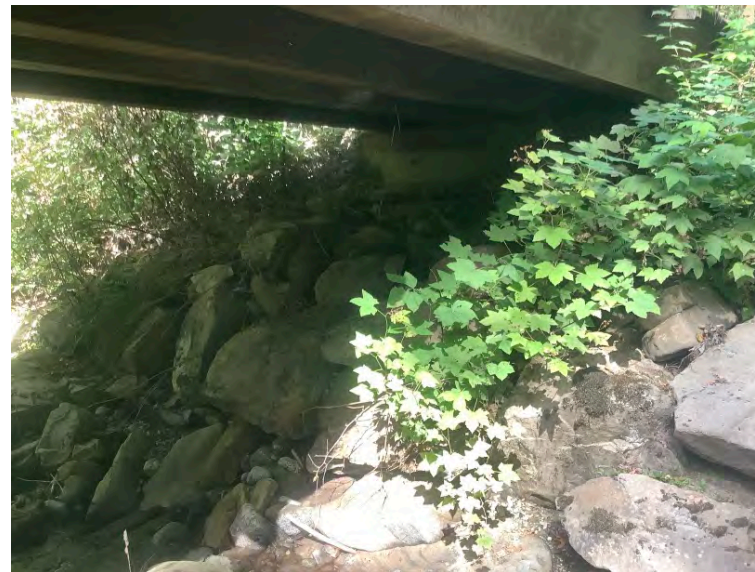
Right Bank Abutment when facing downstream
