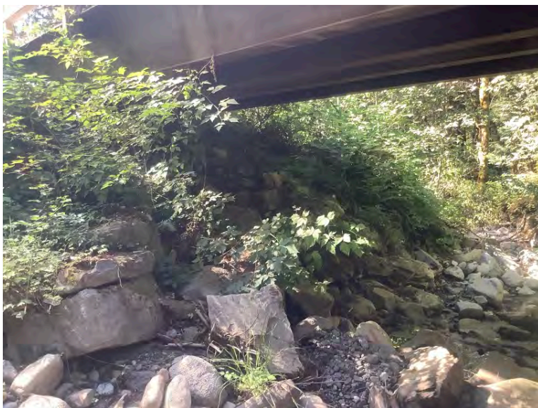
Left Bank Abutment when facing downstream
